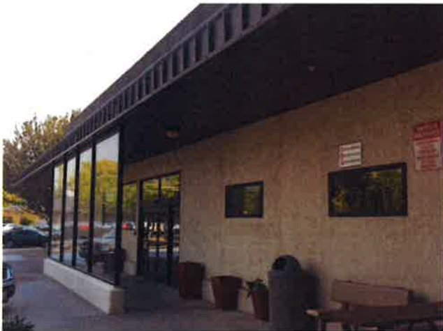
Looking east/front of clinic building
