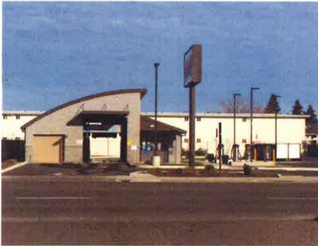
Existing car wash building
