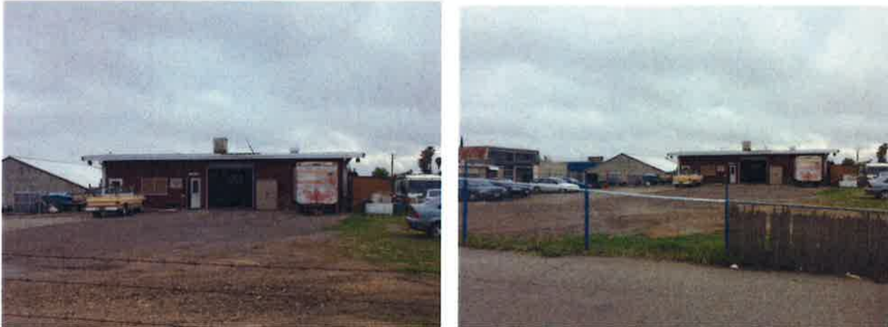
Existing building on project site
