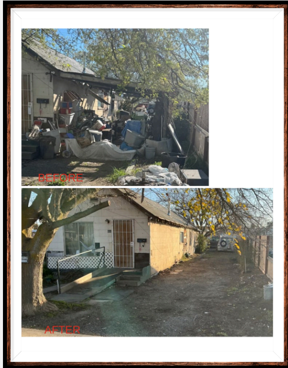
North Butte Street - Before & After
