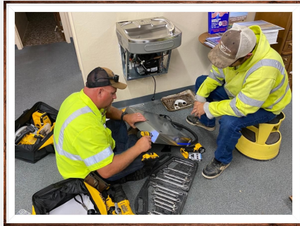
Water fountain Upgrades
