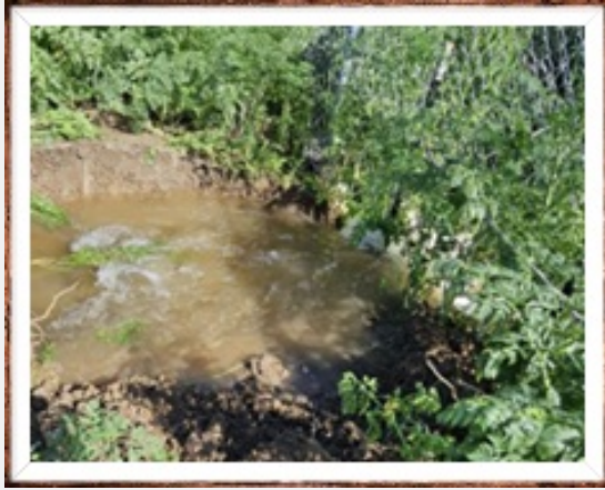
Clogged WWTP drainage ditch.
