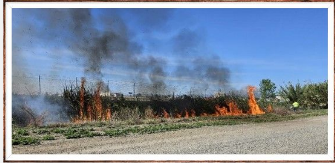
Burning off overgrown vegetation in drainage ditch.
