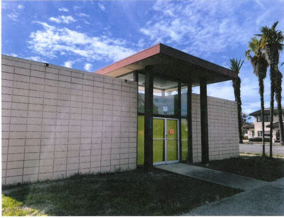
Figure 1 – front of building
