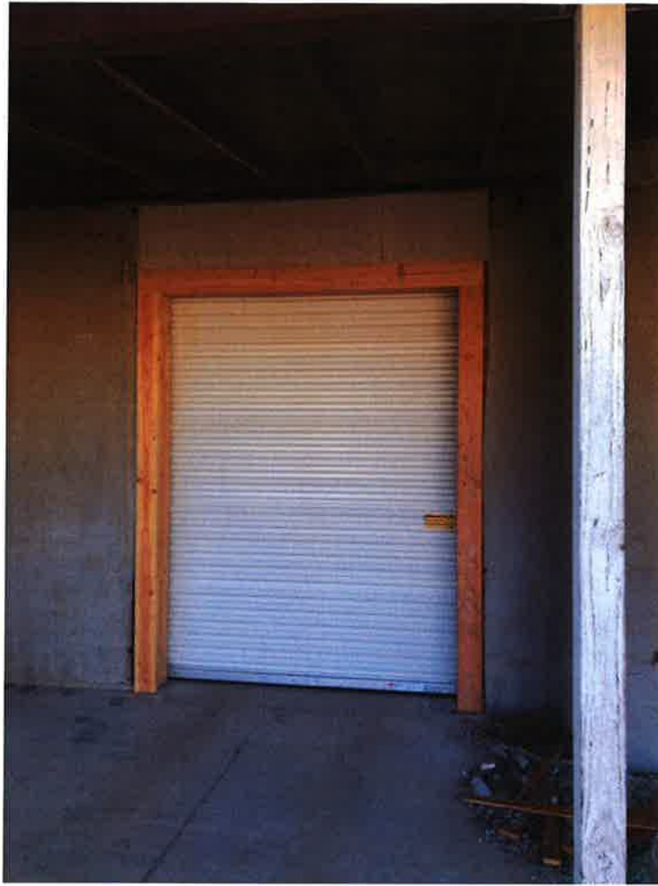
New door installed
