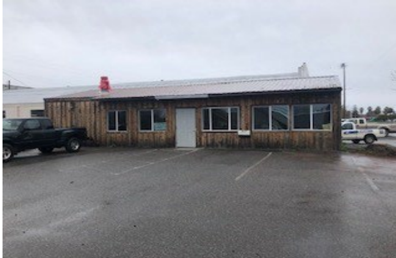
Front of building
